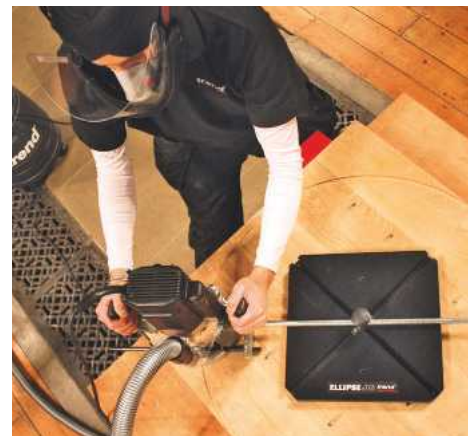
First job involves a router and ellipse jig
